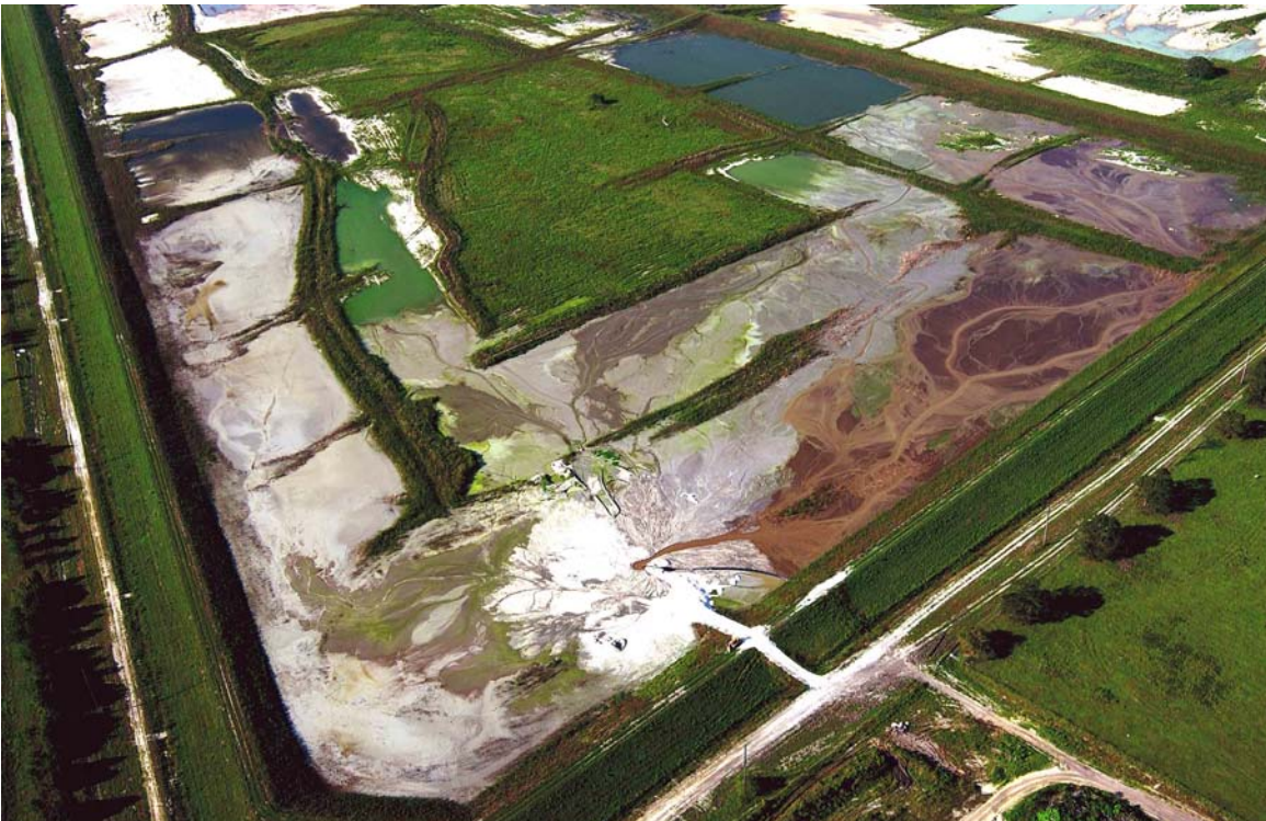
Aerial view of the dredge discharge point at the northeast corner of Settling Cell 1 taken October 4, 2004
