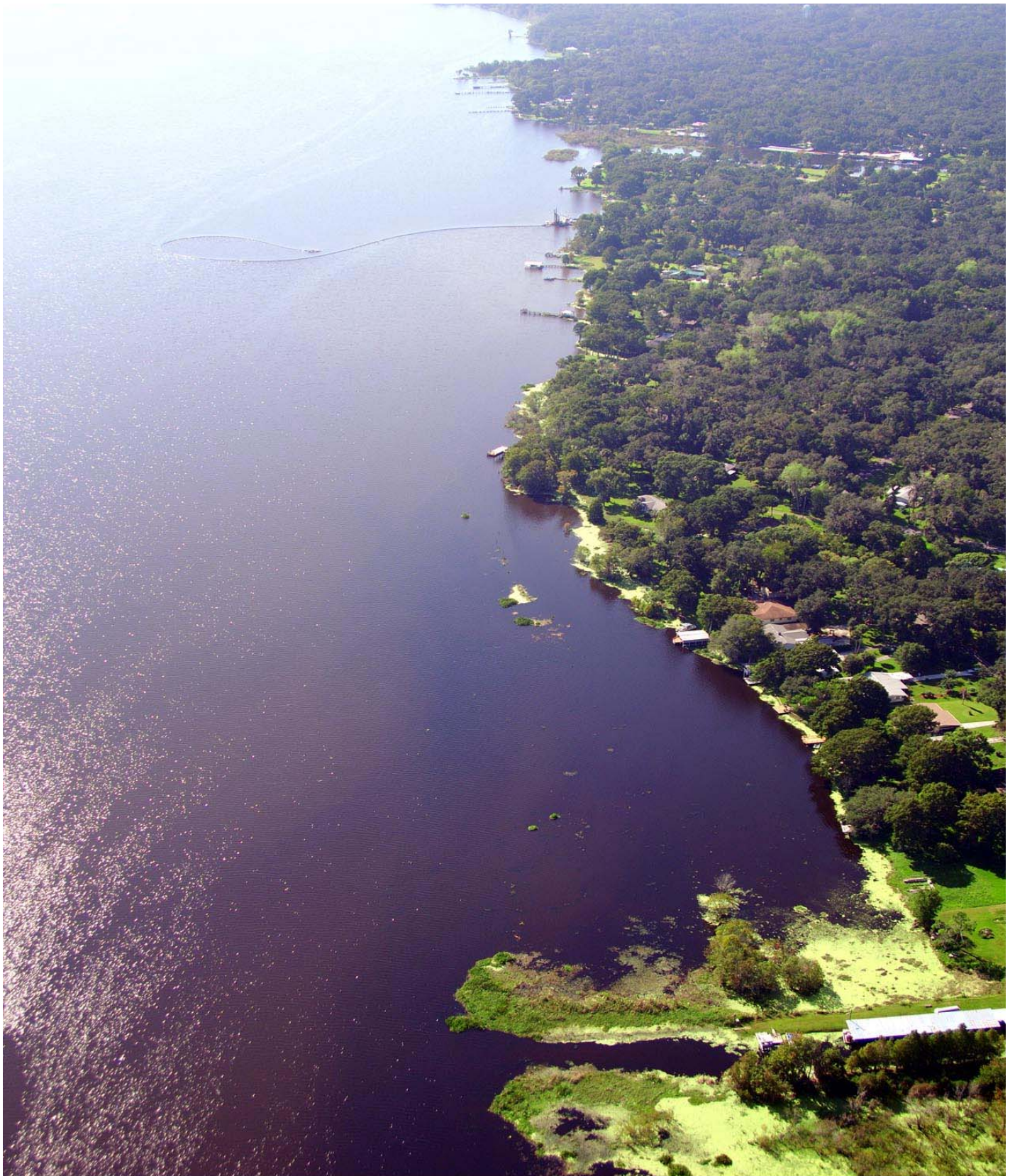
Figure 15 - The western shoreline of Lake Panasoffkee immediately south of Idlewild fish camp after being cleared by the cookie-cutter prior to being dredged
